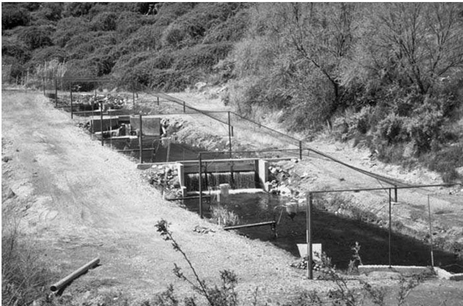
Figure 9.1 An earthen flow-through raceway.
