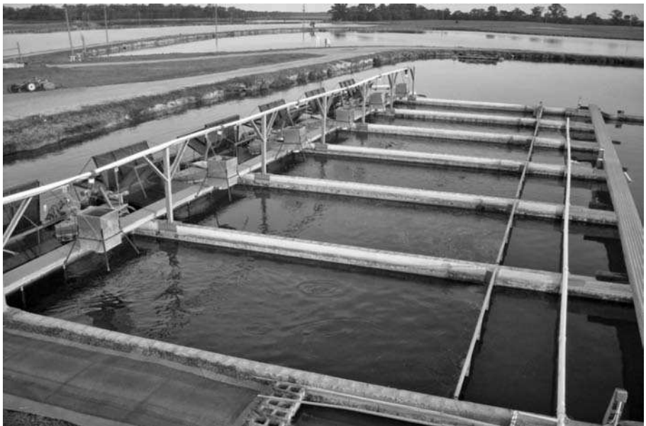
Figure 13.13 Alabama in-pond raceway system.
