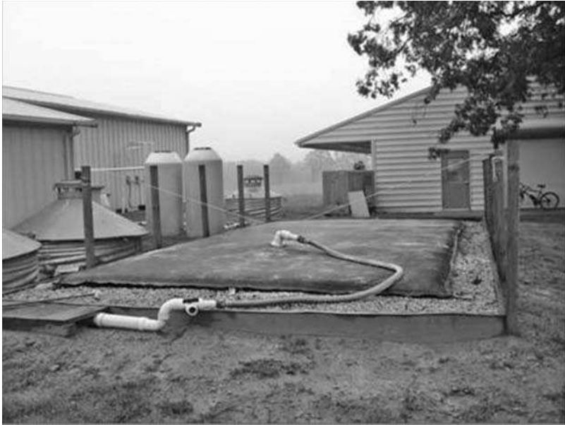
Figure 11.4 Geotextile bag on gravel bed designed to capture leached water for reuse.
