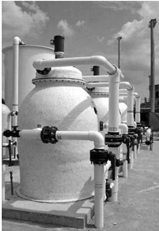
Figure 11.5 Propeller washed bead filter for biofiltration and solids capture.
