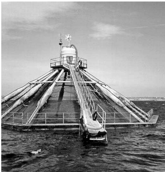
Figure 7.7 A photo of the modified gravity cage system developed by Farmocean International of Sweden. The top center component of the structure is the built-in feeding system.
