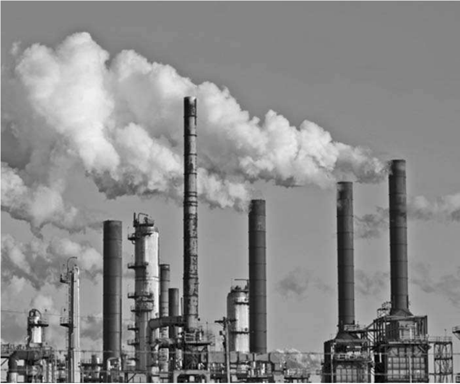
Figure 16.6 A coal-fired power plant.
