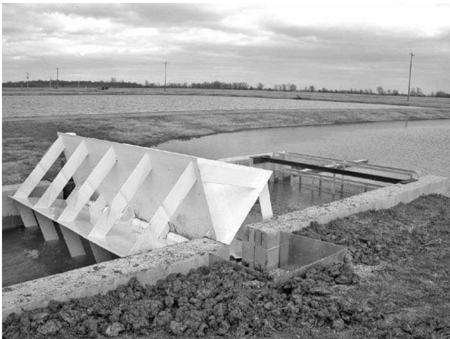
Figure 13.15 Paddlewheel at Mississippi split-pond levee.
